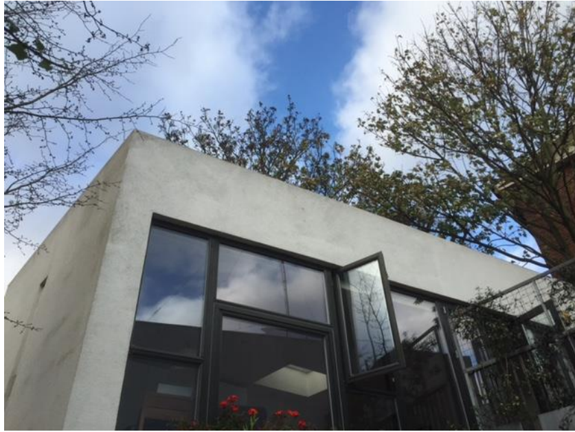
Image 5: View looking up at no. 4
