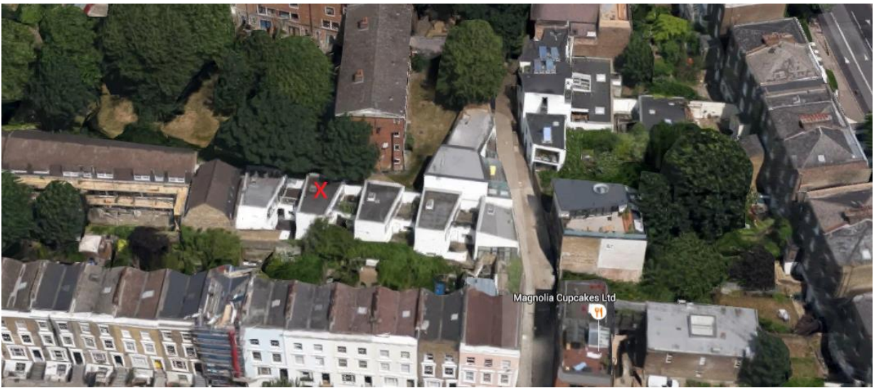
Image 2.: Looking into the site in a Northerly direction
