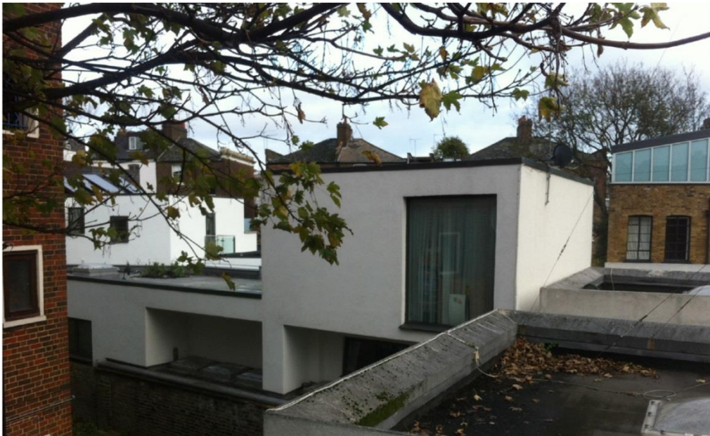
Image 8: View towards first and second floor windows of 37L Mildmay Grove North from flat roof of 4 Colony Mews
