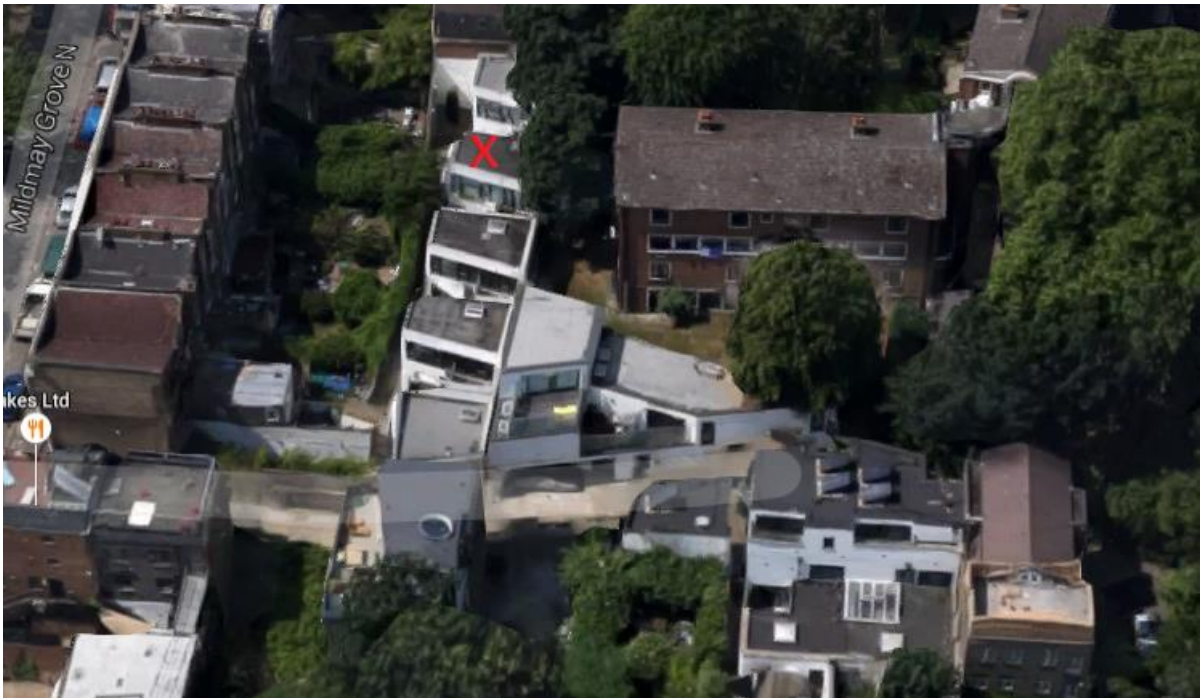
Image 4: Looking into the site in a westerly direction.
